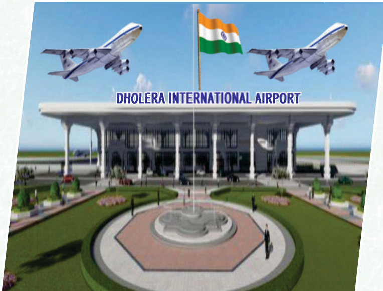
Dholera International Airport
